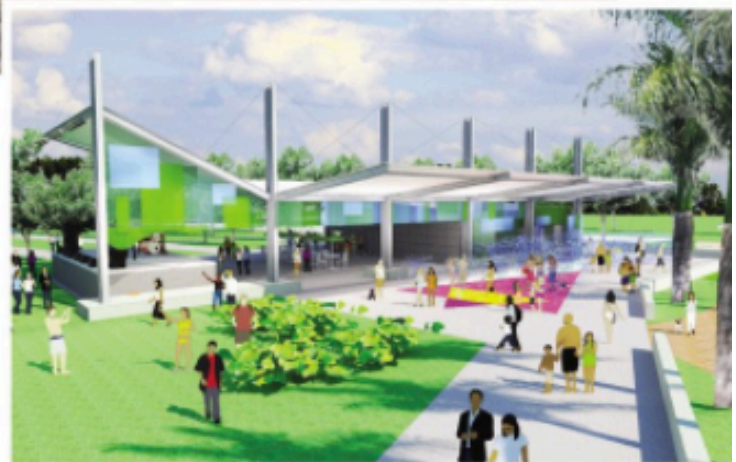
The Riviera Beach waterfront village project, which is expected to open this spring, includes the Marine Events Center (construction pictured above), as well as the Bicentennial Park (rendering above).
